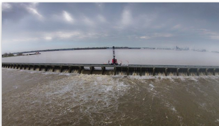
Bonnet Carre Spillway floodwaters release.
